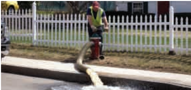
John Leach performing bi-annual water main flushing
